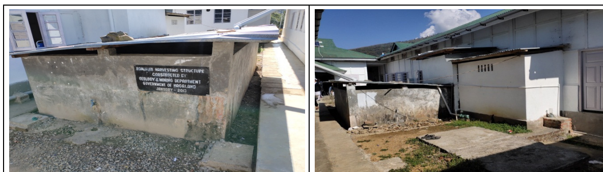
Photograph 5.18: Water storage tanks in DH Wokha
